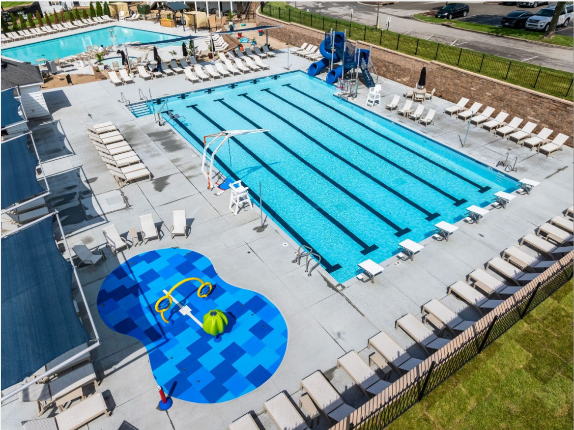
2024 Full renovation of Olympic Pool
